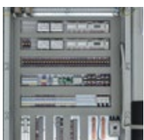
4 Full cabling, including control panel and controller specifically designed for the unit
